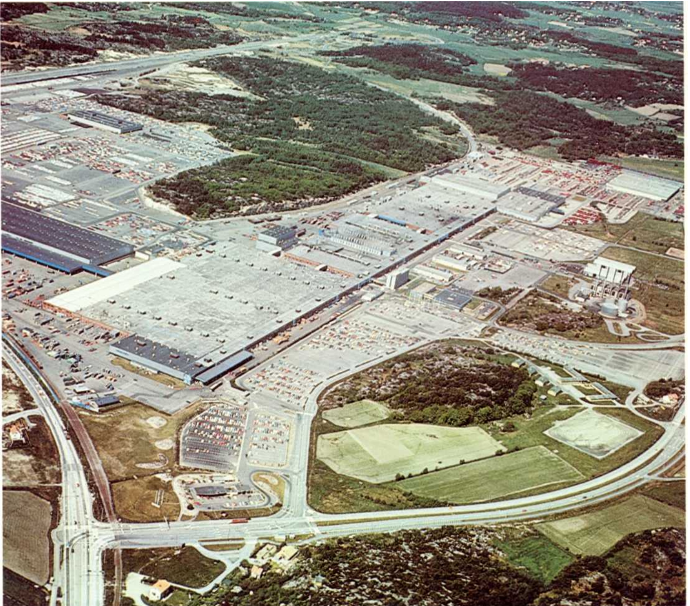
The Volvo Torsslunda Plant in Gothenburg is Volvo's largest facility. The Volvo 240/260 Series are manufactured and assembled here. Volvo has car assembly plants in nine countries.
